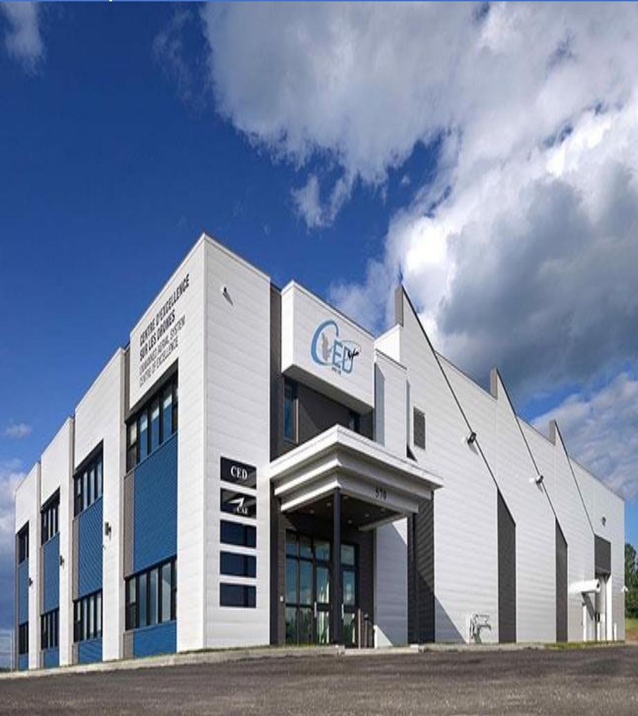
UAS CE main building.
